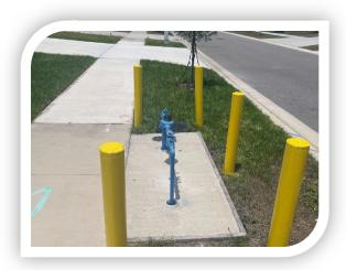
Leaking irrigation backflow was repaired.
