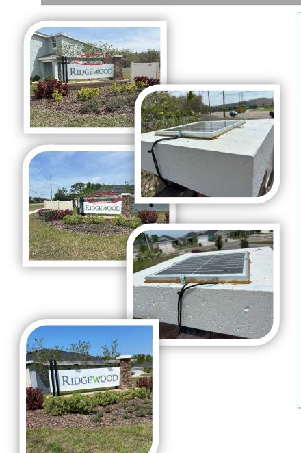
All (3) solar powered monument light fixtures have been installed in Ridgewood – North. Panels were installed flat on the topper of the monument column and reinforced with brackets and hi-strength adhesive.
